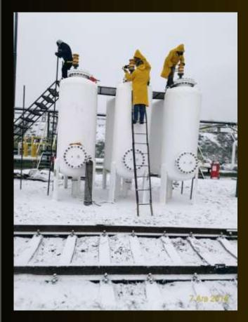
In order to reduce the sulphur content of LPG for very specific purposes such as to use in propellants in cosmetics sector; or to use in gas mixtures that are used to inflate isolation foams in building materials industry; or in refrigerants in white goods sector, these special tanks utilise very specific minerals. Purified output provides corrosion and exhaust emissions less than 6 m/nm³. Single or twin tower, serial or parallel versions are available.
